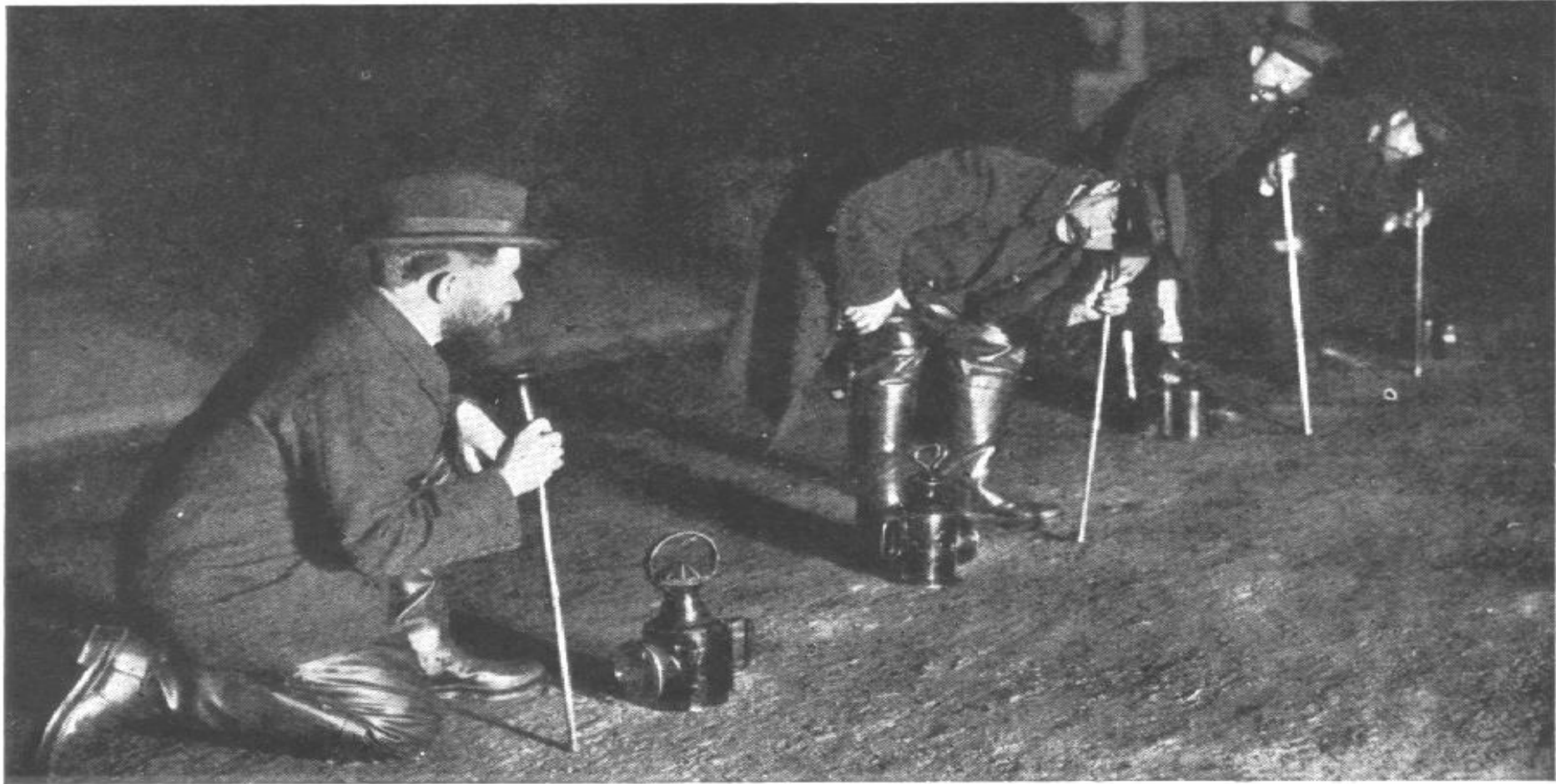
LISTENING WITH STETHOSCOPES AND AQUAPHONES ALONG A MAIN SUPPLY PIPE DURING A NIGHT INSPECTION.
