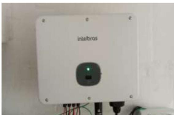
**Figura 3** – Inversor On-Grid 20kW EGT 20000 MAX (380V) (Intelbras)
